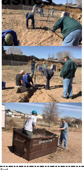
The radial wire crew buried ~1000-ft of radial wires radiating like spokes from the new antenna.
