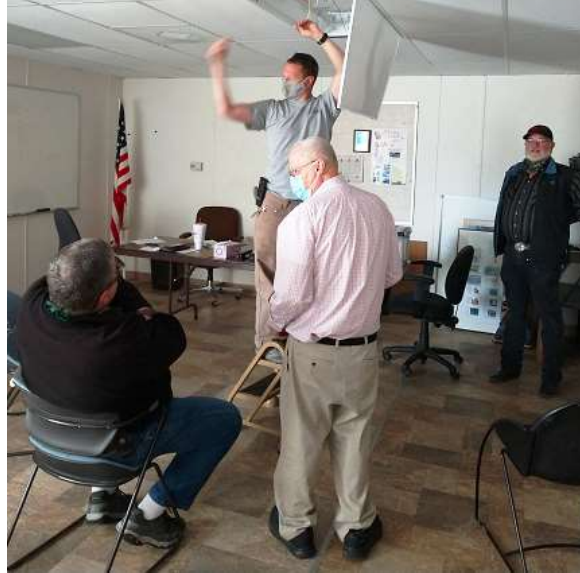
Repairs at the clubhouse!
