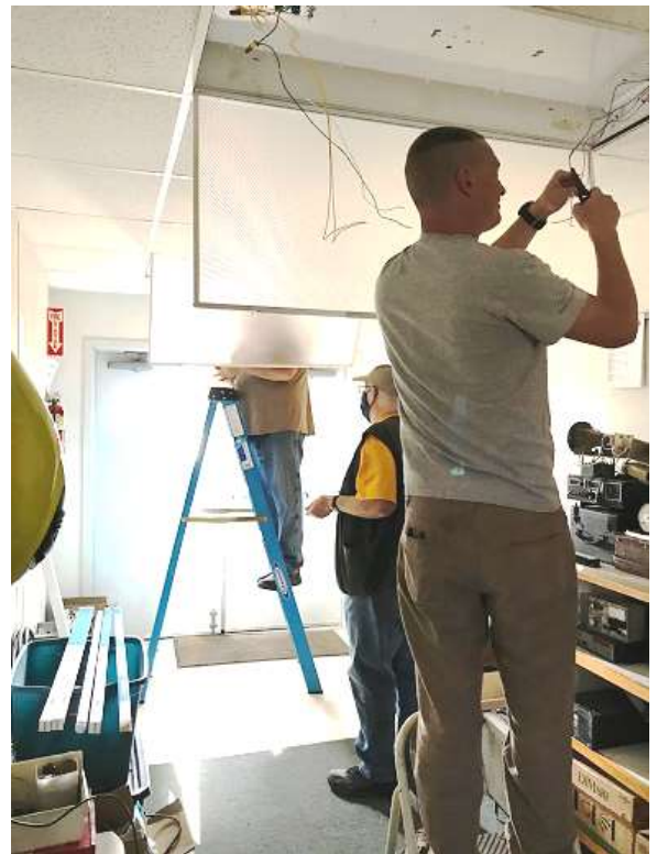
Repairs at the clubhouse!
