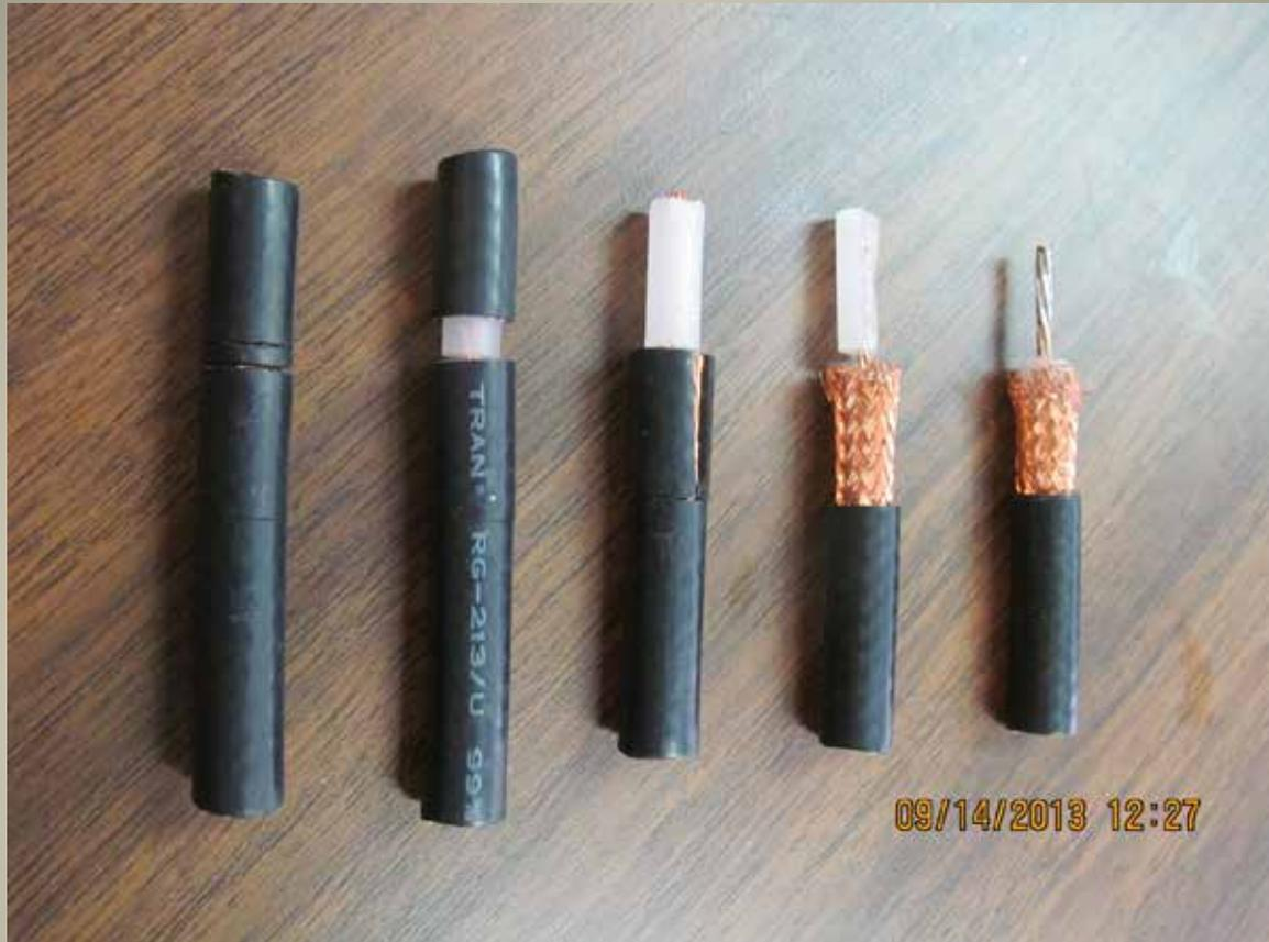
The evolution of a connector installation (note one is out of order).
