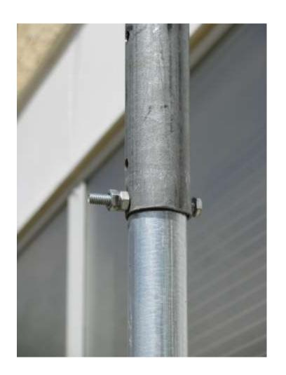
The mast assembly is supported by a clamp attached to the roof peak.
